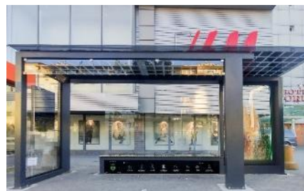
Fot 9 Smart Bus Stop
